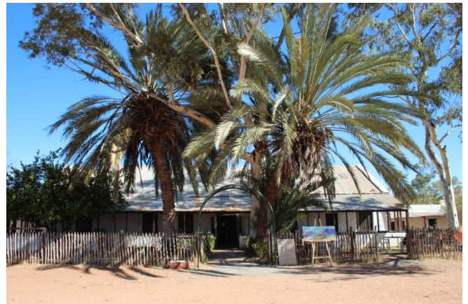
The Strehlow's House and now cafe
