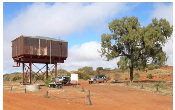
This was the old water tank back in 2010
